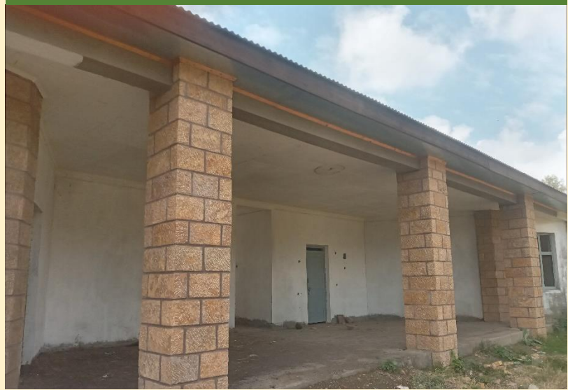
Kindergarten building March 2023
